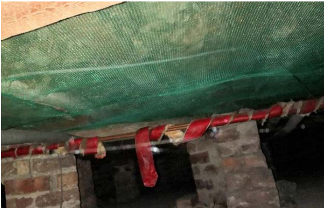
Insulation secured to the underside of floorboards
